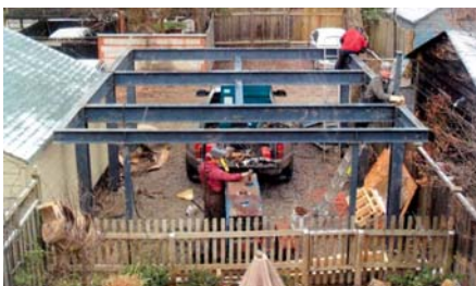
Installation of steel I-beam construction.
