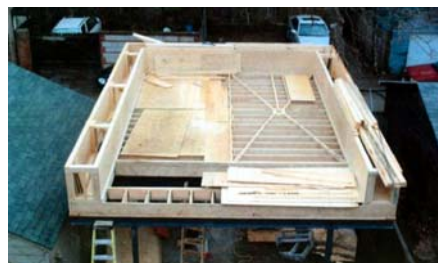
The roof and planter are created with wood frame construction.
